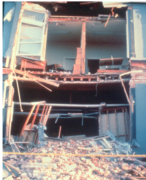
Figure 22.7 Unsupported Bearing Walls
