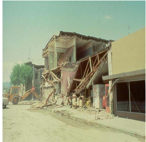
Figure 22.1 Light-Frame Collapse
