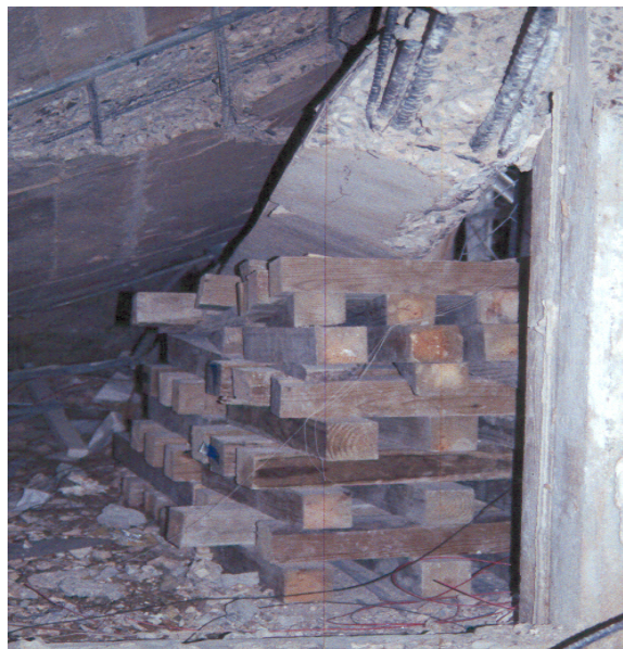
Figure 22.21 Sloped Surface Shore with Cribbing
