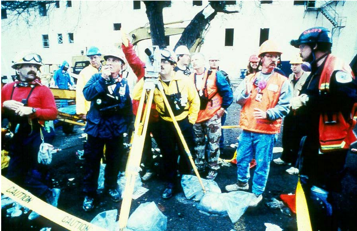
Figure 22.9 Monitoring a Collapse
