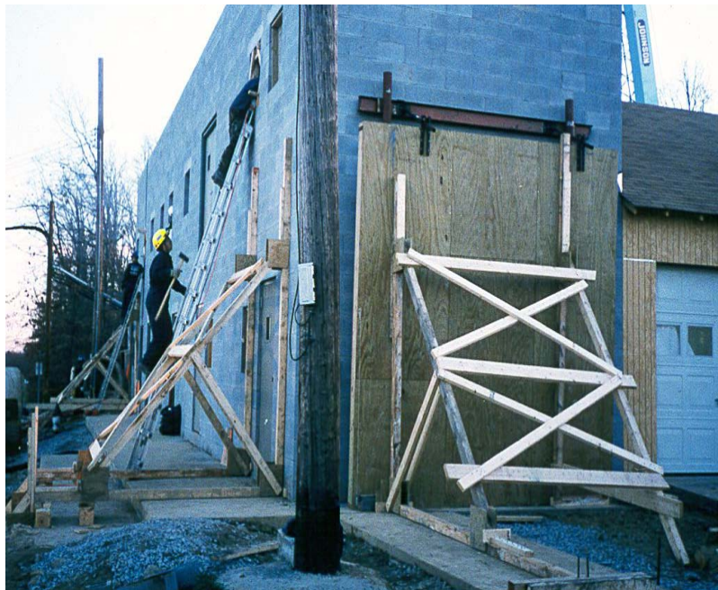
Figure 31.1 Raker Shores
