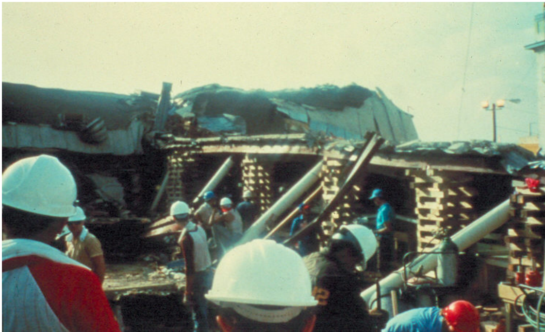
Figure 30.1 Sloped Floor Shoring
