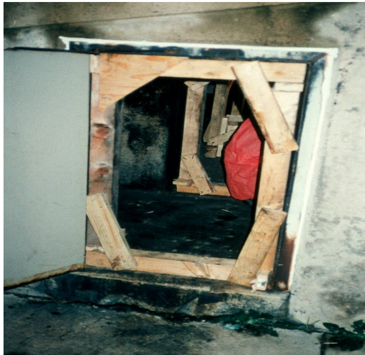
Figure 29.1 Window and Door Shore
