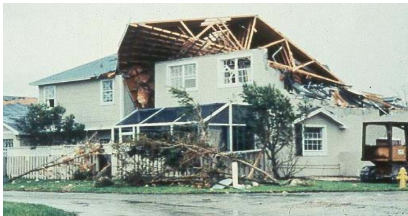
Figure 22.3 Light-Frame Collapse
