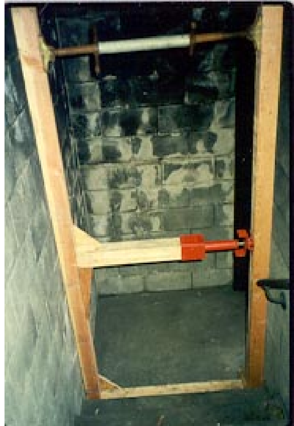
Figure 28.1 Horizontal Shore
