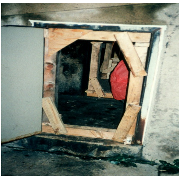
Figure 22.20 Window and Door Shore
