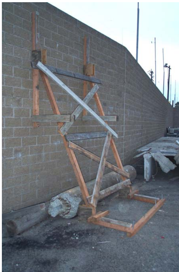
Figure 31.2 Flying Raker Shore
