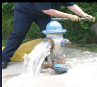
Step 5: Open the hydrant enough to verify flow and flush hydrant. (Dry-barrel hydrant only.)
