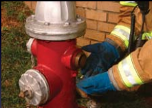
Step 3: Leave one hydrant outlet open until the hydrant is fully drained.
