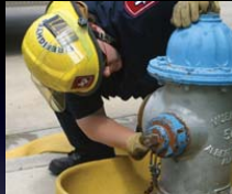
Step 2: Quickly look inside the hydrant opening for foreign objects. (Dry-barrel hydrant only.)
