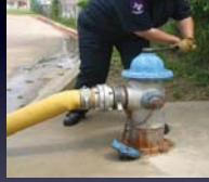
Step 8: When instructed, turn the hydrant wrench to fully open the valve.
