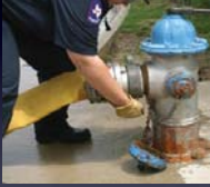
Step 7: Attach hose or valve to the hydrant outlet(s).
