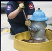
Step 3: Check to ensure that the remaining caps are snugly attached. (Dry-barrel hydrant only.)
