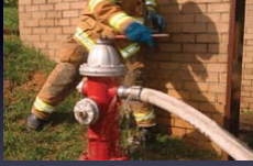
Step 1: Turn the wrench to slowly close the hydrant valve.
