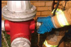
Step 4: Replace the hydrant cap.
