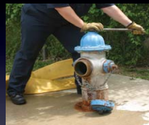
Step 6: Shut off the flow of water. (Dry-barrel hydrant only.)
