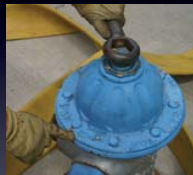
Step 2: Attach the hydrant wrench to the stem nut. Check for an arrow indicating the direction to turn to open.
