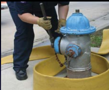
Step 1: Remove the cap from the outlet you will be using.
